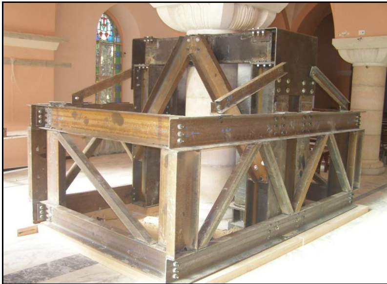
Photo 3. The shoring steel frame
