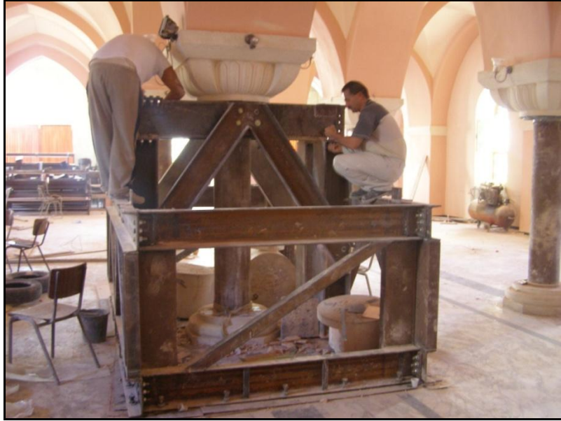
Photo 4. The Shoring Steel Frame
